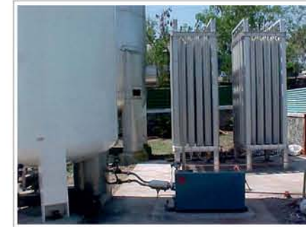
High Pressure Vaporiser For Cylinder Filling
