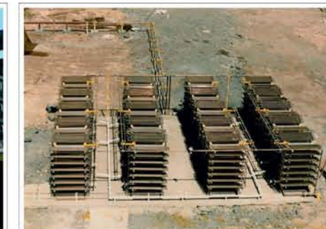
4000 Nm 3 / Hr All Copper Vaporizer Built In 1989
