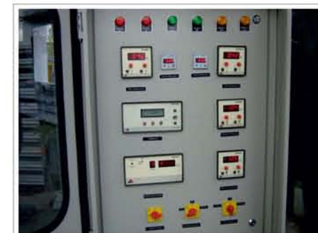
Automatic Control Panel and Switch over skid for 24 x 7 unattended vaporiser operation
