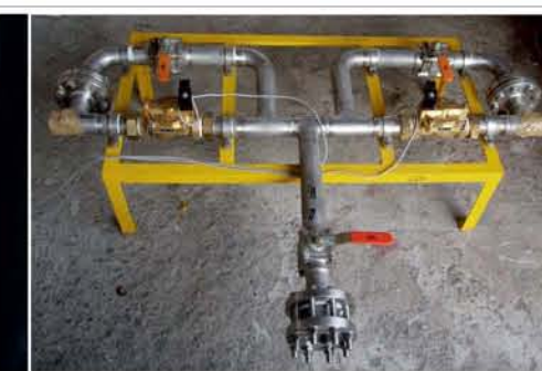
Automatic Control Panel and Switch over skid for 24 x 7 unattended vaporiser operation
